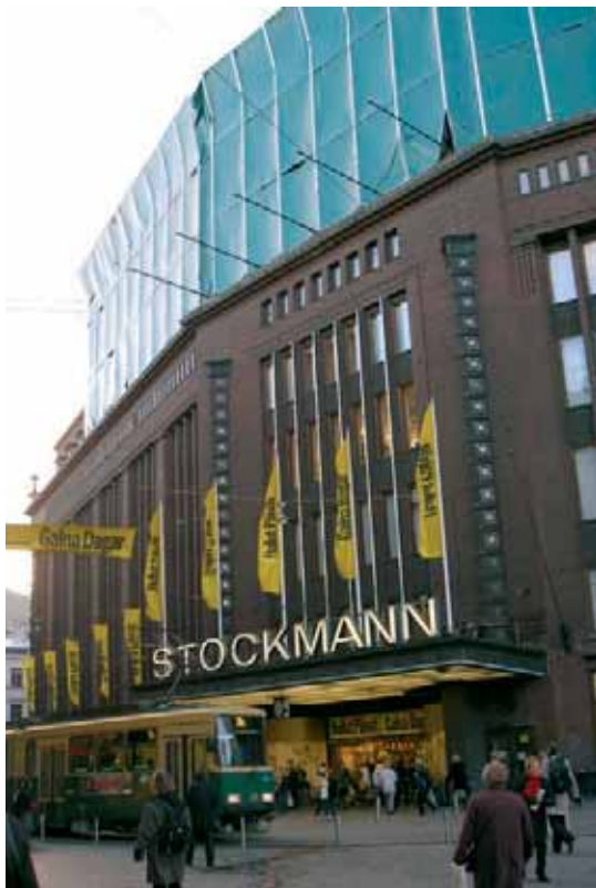
The warehouse Stockmann in Helsinki (under reconstruction); Source: Anna Nurmi
